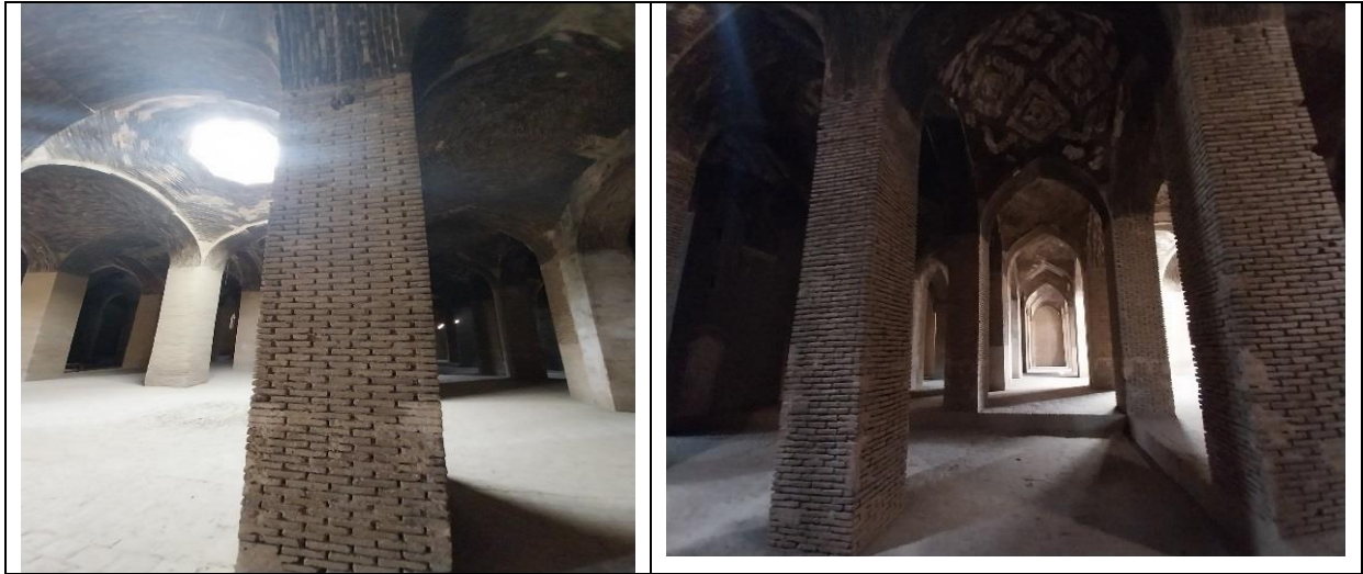
Figure 15. Images of inner courtyard, ceiling, columns (photo, from the author's archive)
