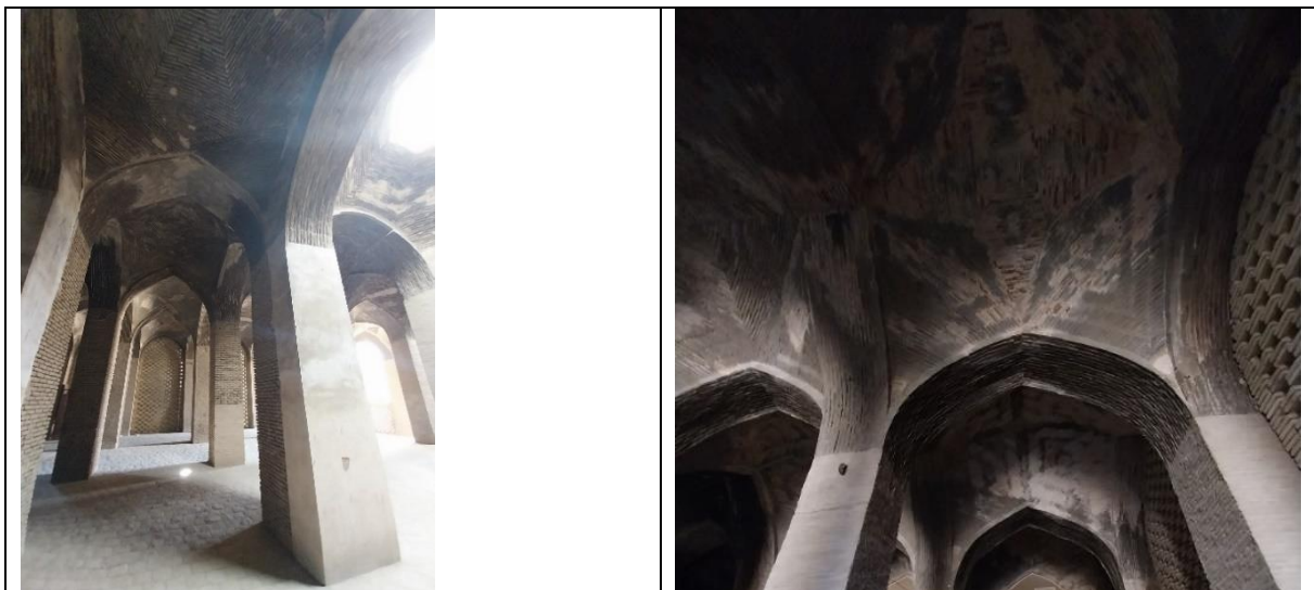
Figure 14. Images of inner courtyard, ceiling, columns (photo, from the author's archive)
