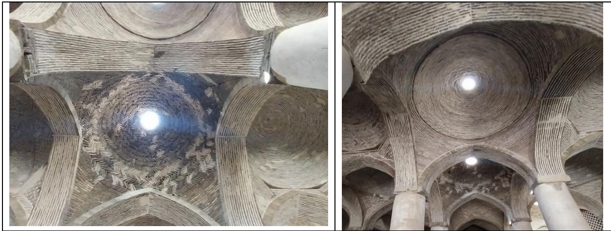
Figure 21. Images of inner courtyard, ceiling, columns (photo, from the author's archive)
