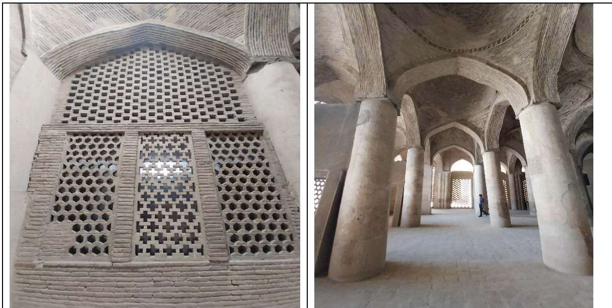
Figure 16. Images of inner courtyard, ceiling, columns (photo, from the author's archive)
