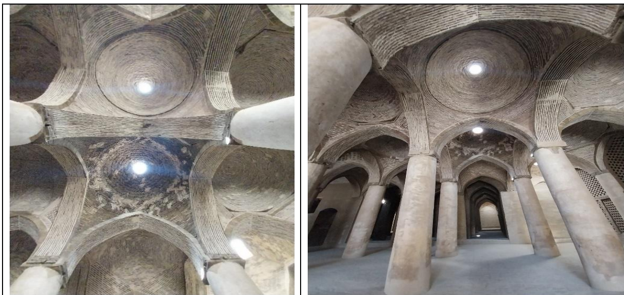
Figure 20. Images of inner courtyard, ceiling, columns (photo, from the author's archive)
