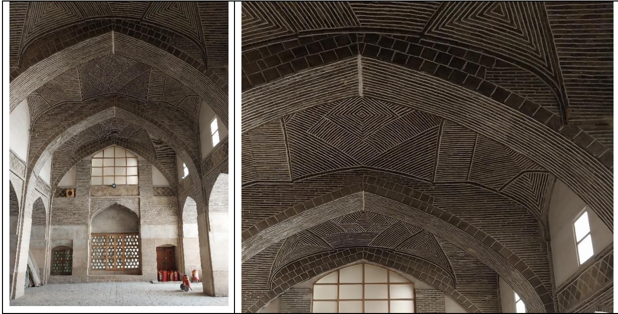
Figure 17. Images of inner courtyard, ceiling, columns (photo, from the author's archive)
