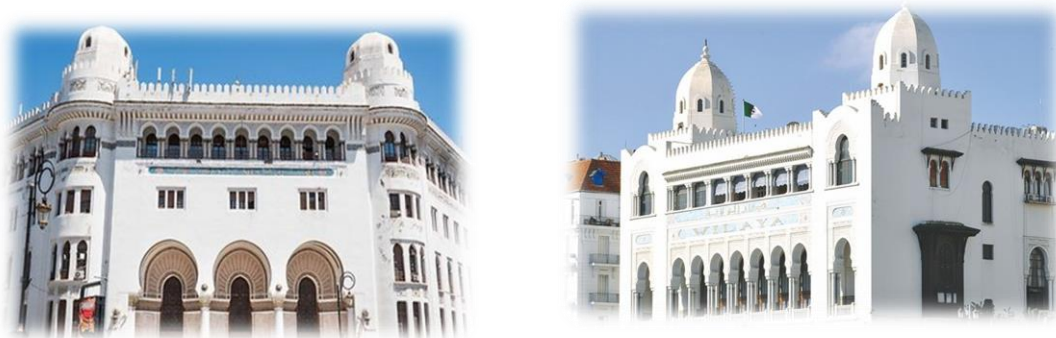
Figure 3. Great Post Office (left), headquarter of Algiers prefecture (right), two public buildings expressing the colonial neo-Moorish style.
