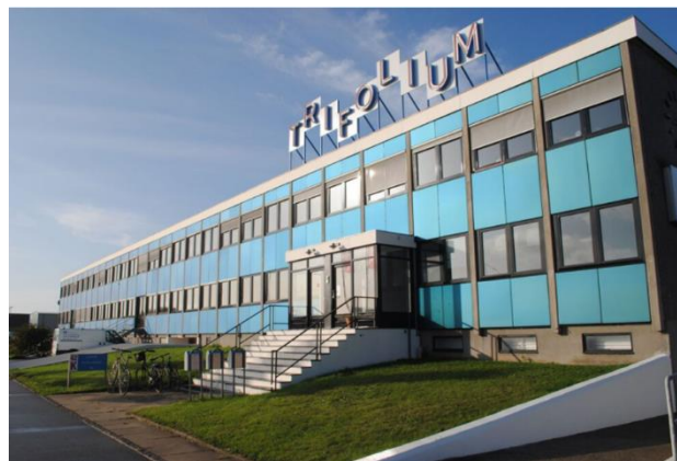
Fig. 5. Trifolium Office showing the distribution of glazed solar thermal collectors in bluish green [16].
